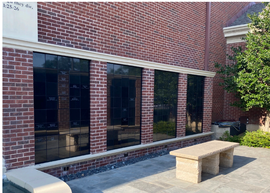
SIMILAR NICHE INSTALLATION (CUSTER ROAD UNITED METHODIST CHURCH)
