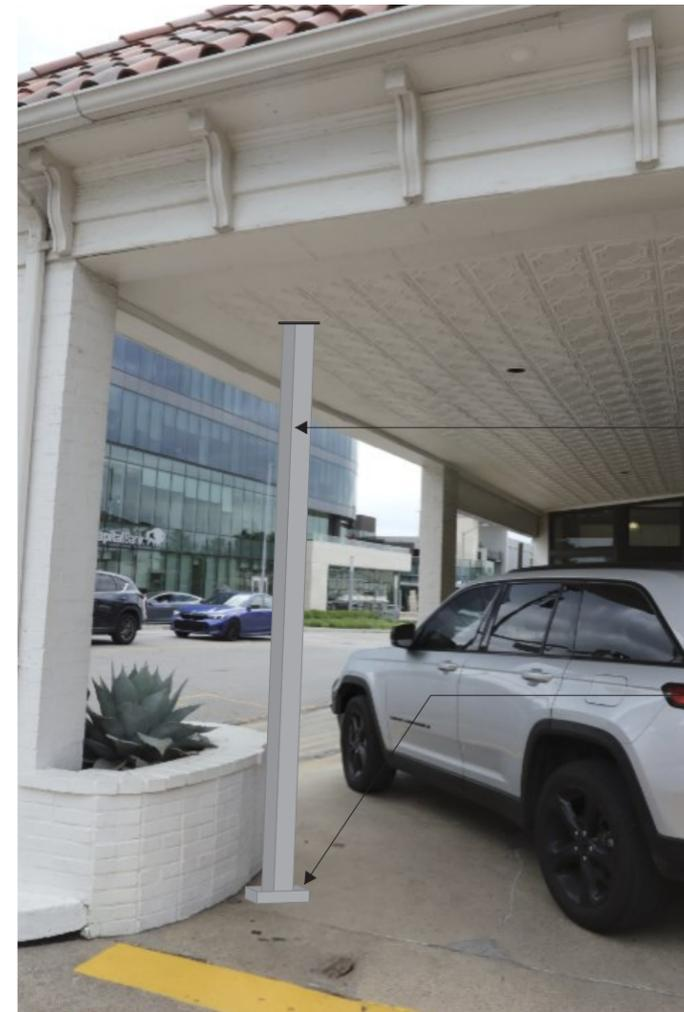
4"x4" STEEL TUBE UNDER CANOPY & INTO ROOF PAINTED WHITE
